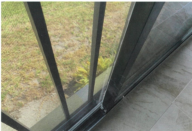
Balcony Floor Tile
