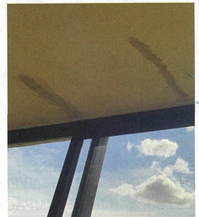
Unpainted Crack Repairs
